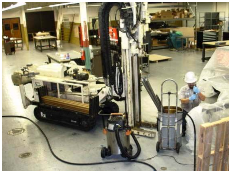
Photo 1 Injections Inside the Facility
