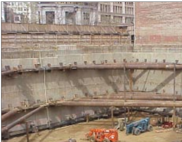
Excavation in Progress
