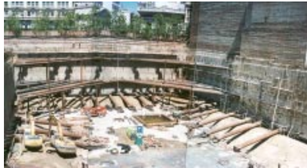
Level Three Bracing - Northerly View
