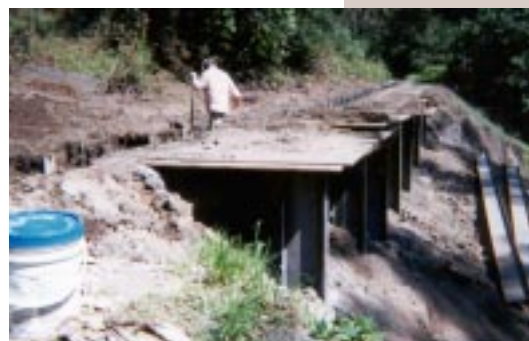
Figure 3 Thirty-four permanent piles were installed south of buried pipeline.
