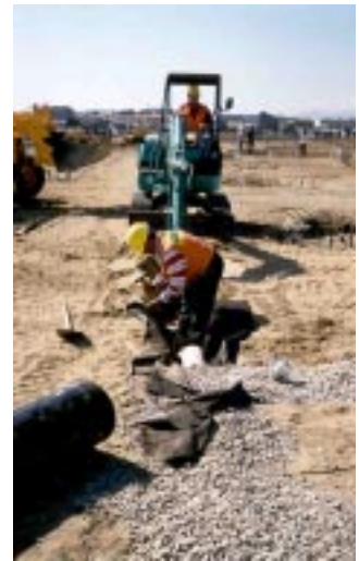
Installation of Methane Collection Piping
