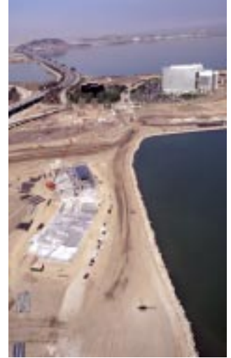
Sierra Point (1999) The 131-acre development with site preparation and construction in progress simultaneously. The view is northward along Highway 101 with Candlestick Point and Hunter's Point in the far background.
