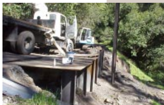
Figure 2 Temporary soldier piles provided temporary support for vehicle access.
