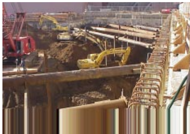
Excavation for Level Two Bracing
